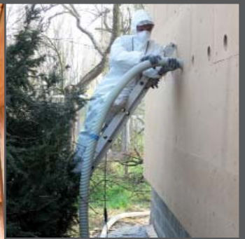
Insufflation de l'isolation
